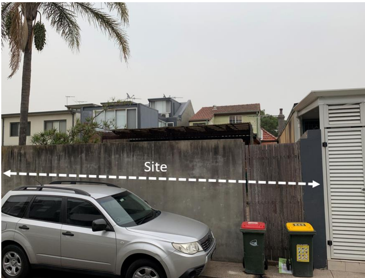
Figure 3: Rear of site viewed from Salisbury Lane.
