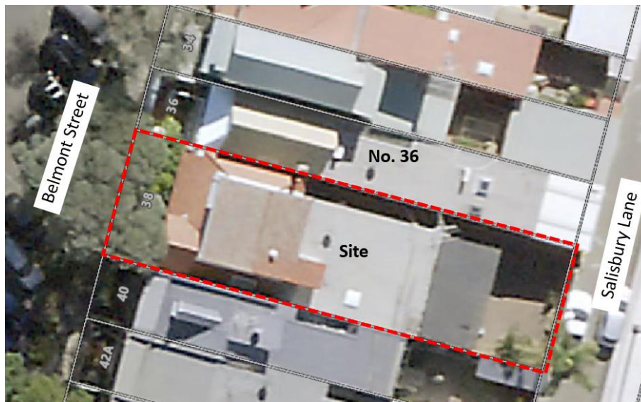
Figure 11: Aerial photograph of the site and the adjoining dwelling at No. 36.
